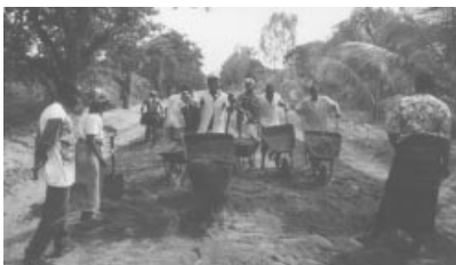
Local workers spreading gravel, Mozambique
