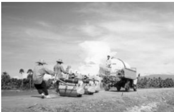
Compaction of gravel surface, Kampot Province
