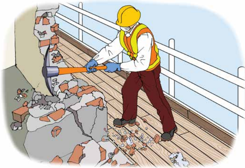
Figure 36.1. A scaffold platform from which demolition may be carried out safely. Manual demolition should be planned before starting the work. Workers should receive detailed instructions on the working process, as well as the hazards and risk prevention measures.
