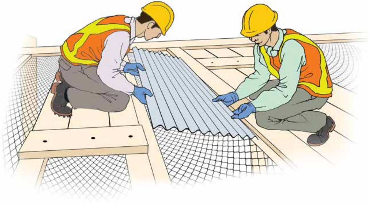
Figure 10.1. Installing horizontal safety nets is a good additional measure to minimize the effect of a fall, in the event that the primary measures prove to be inadequate.
