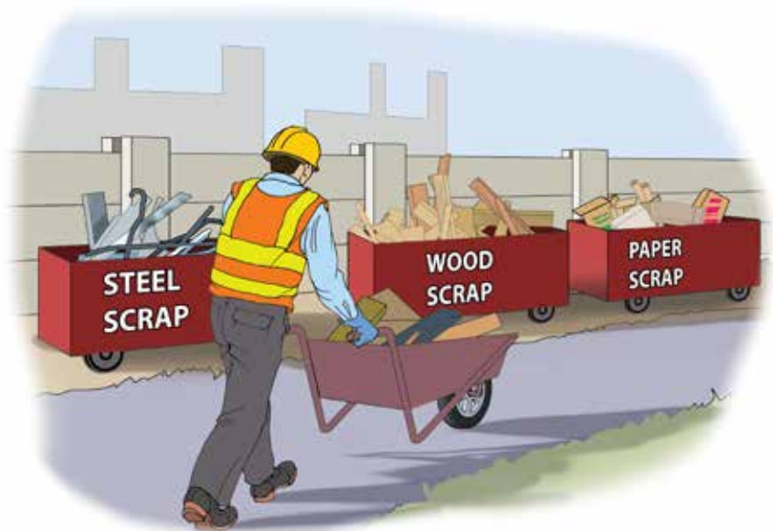
Figure 3.3. Place containers near the transport passageways for the collection of unnecessary materials.
