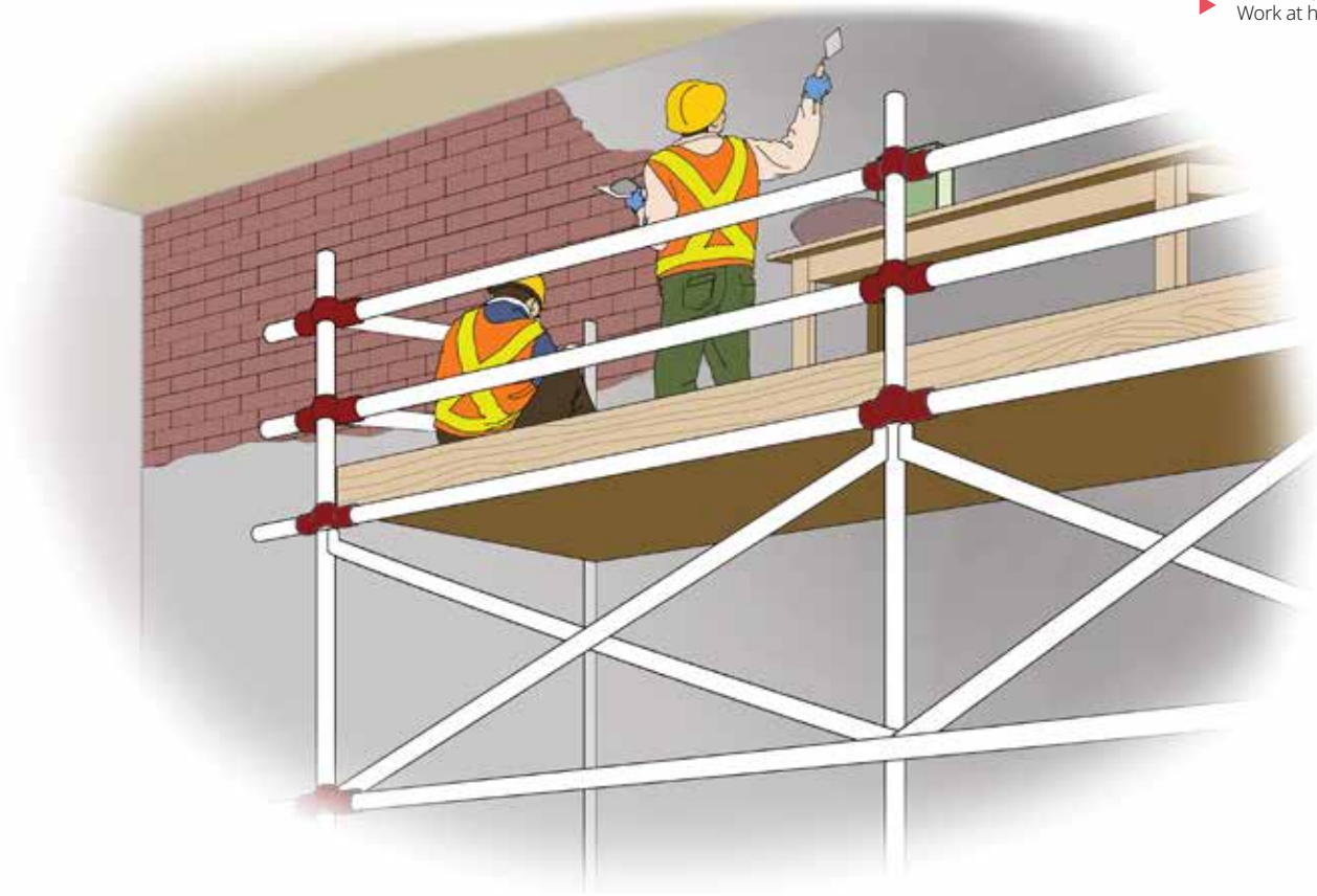
Figure 8.1. Bring only the tools and materials needed for immediate use and evenly distribute the materials over the scaffolding to avoid overloading.
