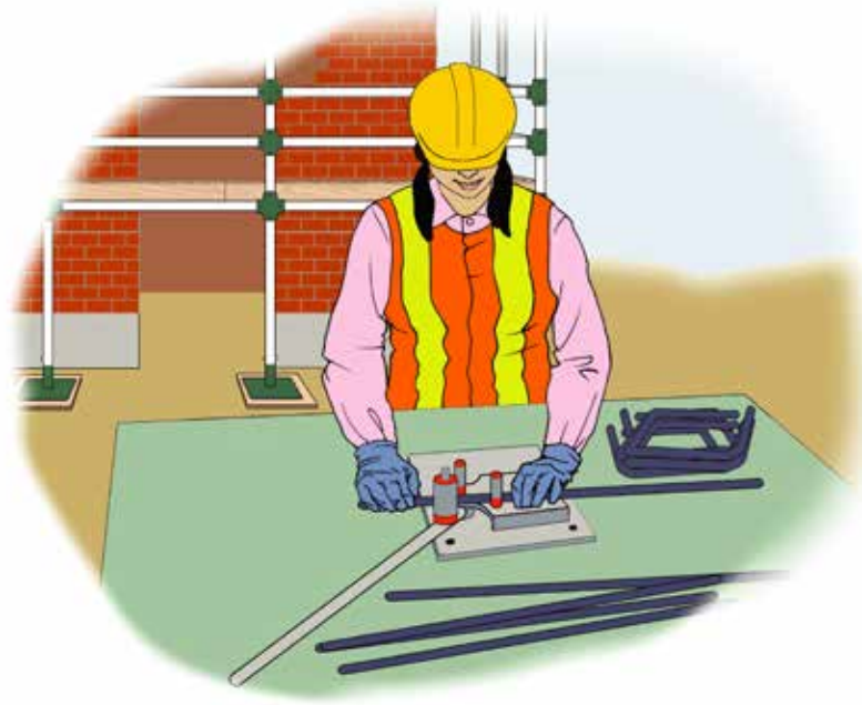
Figure 19.1. Place frequently-used tools and materials within easy reach.
