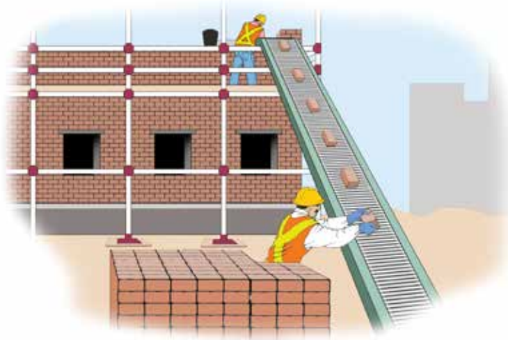
Figure 17.2. Use conveyers to lift a number of bricks and other similar materials.
