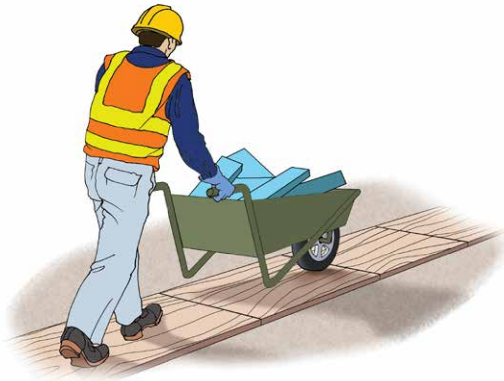
Figure 16.2. Makeshift wood planks used to cover a rough surface on a transport passageway help workers push carts more easily.
