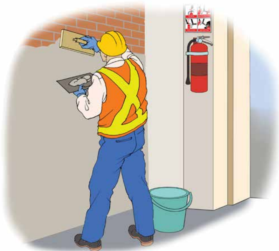
Figure 4.2. Provide that a sufficient number of fire extinguishers are within easy reach and ensure that workers know how to use them.
