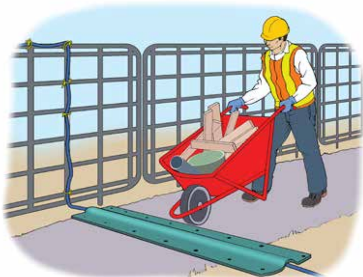
Figure 15.2. Cover electrical wires to ensure electrical safety.
