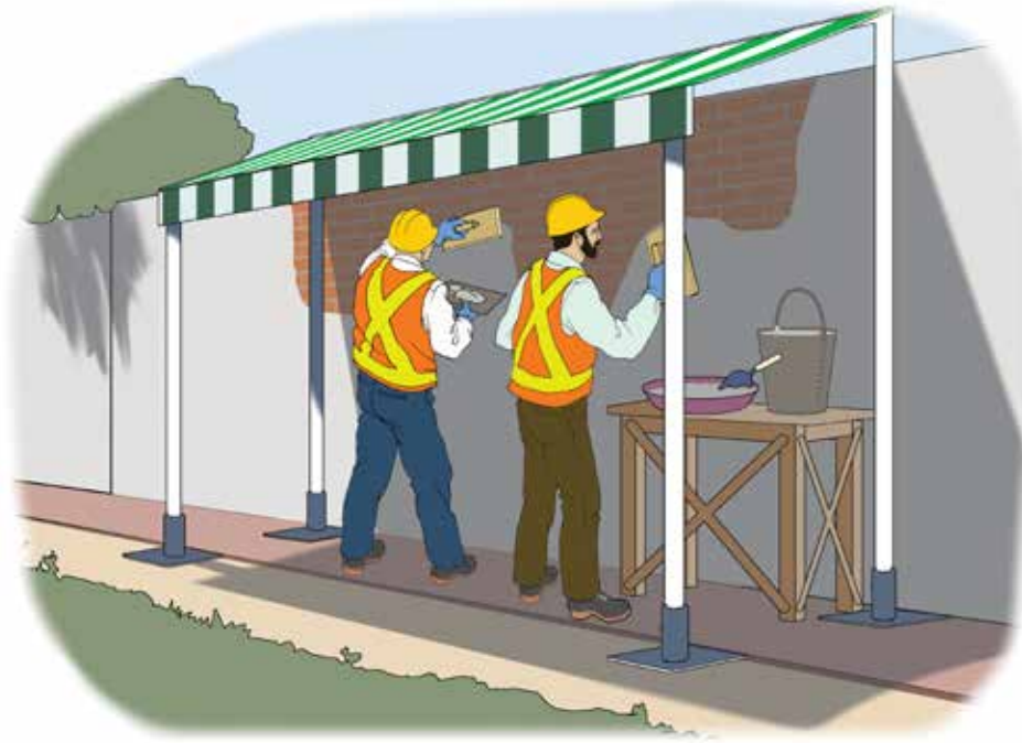
Figure 22.1. Use shades to protect workers from the strong heat of the sun when they are working in open-air environments.
