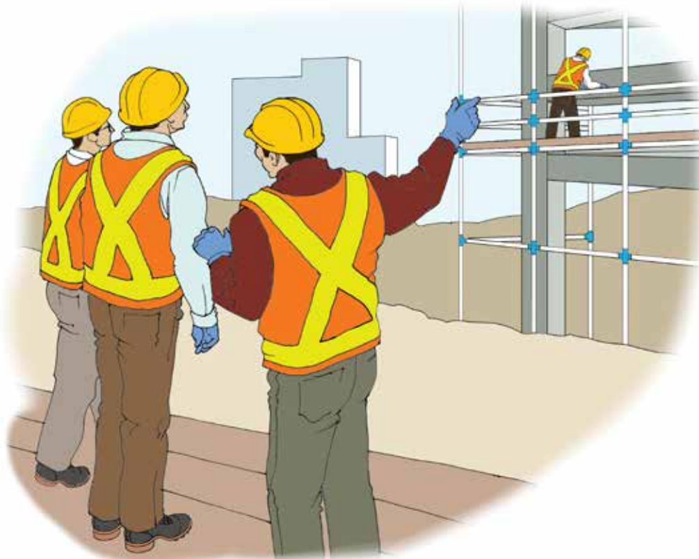
Figure 1.2. Before starting each new activity specified in the schedule, invite workers to jointly analyse the risk prevention measures contained in the SHP. If they are inadequate for the working method envisaged, update the SHP and implement the new measures.
