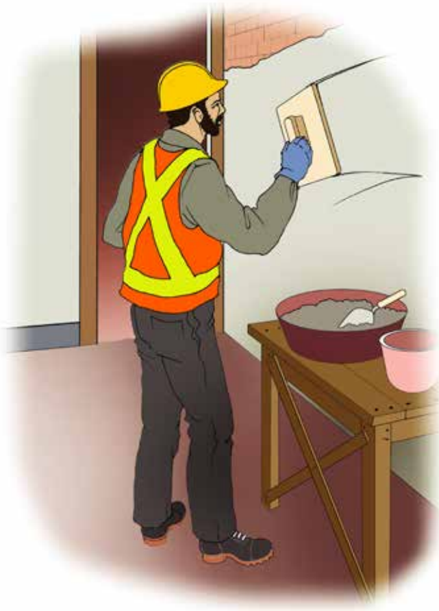
Figure 19.2. Use convenient side workbenches to place necessary tools and materials within easy reach.
