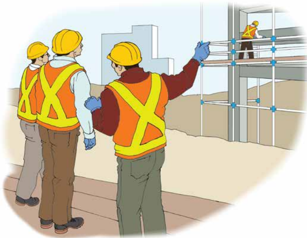
Figure 6.3. After the scaffold has been erected, ask another person to check it all and record all the controls carried out.
