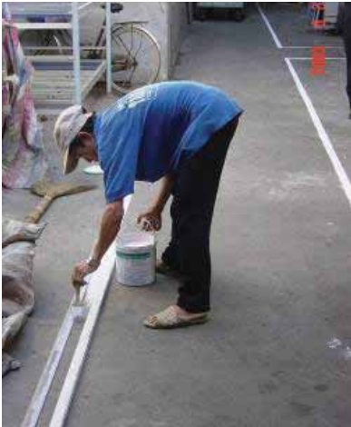
Mark the transport route.
