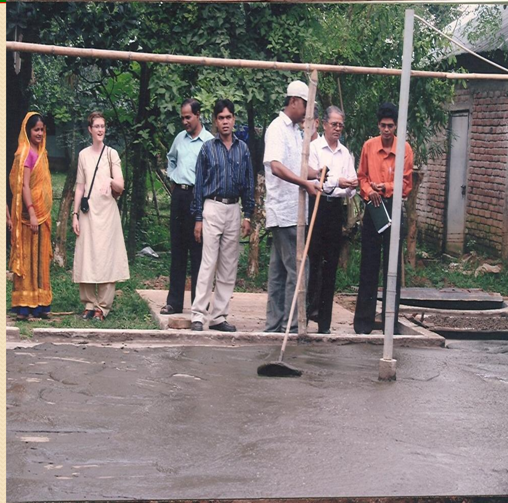
Slurry Processing at a biogas plant
