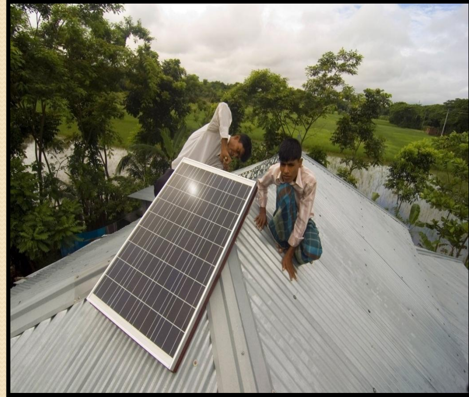
Solar Installation in a rural house
